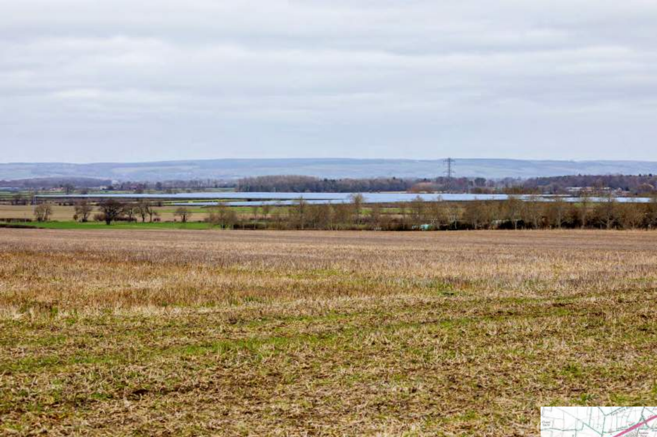
Malton Solar Farm - View 7 - Broughton Road Image 7927
