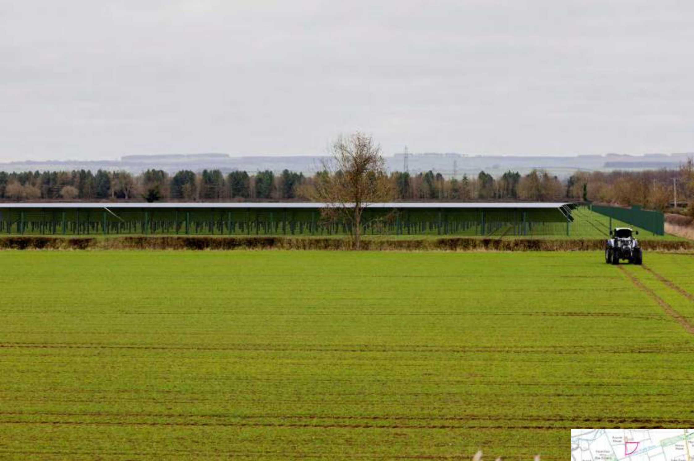
Malton Solar Farm - View 5 - Acomb House Image 7873
